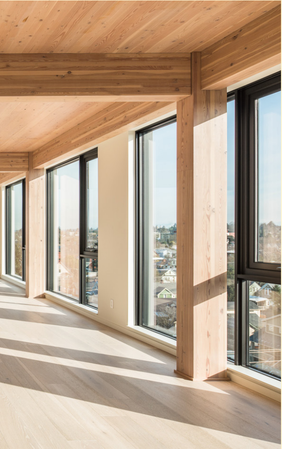
← Carbon 12, Portland, Oregon by Kaiser + Path This 85-foot-high mass timber condo provides residents with modern luxury, sustainable design and state-of-the-art technology. Constructed with sustainably harvested and certified CLT, when it was completed in 2018 it was one of the tallest buildings of its kind in North America, and the project is opening the doors to taller wood buildings throughout the state. (c) Andrew Pogue
