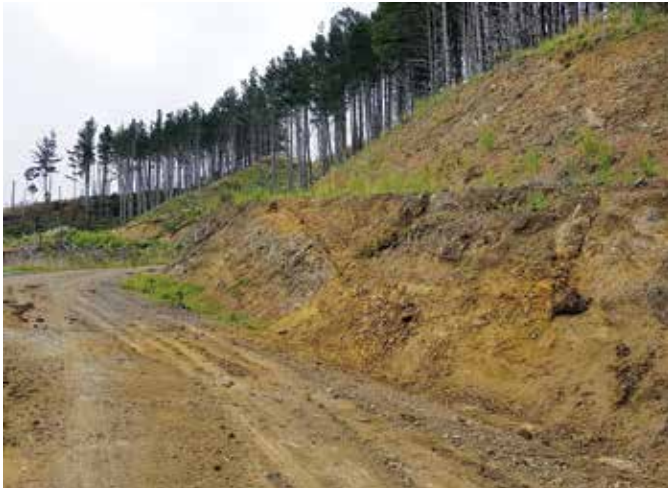
Benched cut slopes
