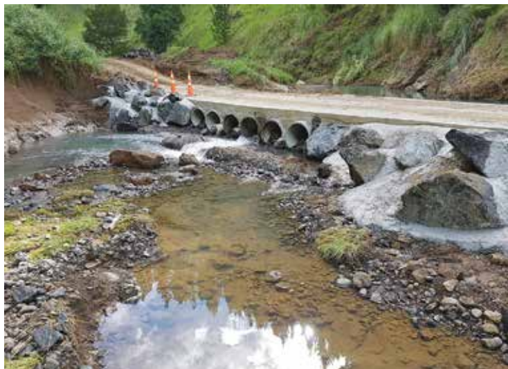
This battery culvert was well constructed, and had relatively minor repairs and maintenance considering the storm flow was 1.5 m above the structure. Left: The reno mattress has protected the crossing from undermining. Note that the gravel movement from the storm has blocked all but one of the pipes. Right: Weaknesses have been armoured. The holes are used to pump grout in and fill the void. Armour known weaknesses
