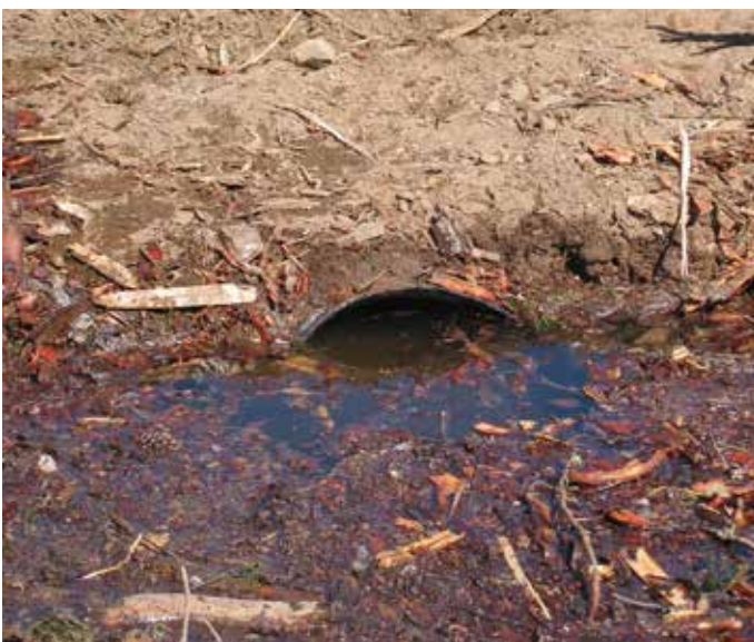
Check for crushed drainage culverts after logging. Drainage culverts are easily damaged if the maintenance operator is inattentive
