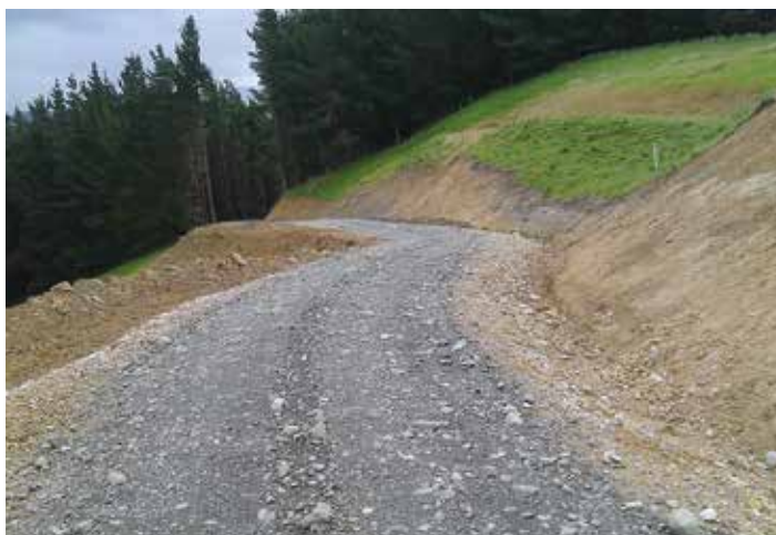
Cut and side cast construction
