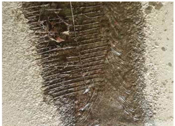
A rusted-through steel culvert floor and a concrete pipe's floor worn past its steel reinforcing
