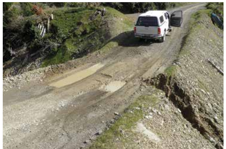
Left: Well-compacted berms were used to protect a large fill slope by directing water away from the more vulnerable earthworks. Water has been directed to cut-outs and flumes on either side of the fill. Right: This large fill is showing failure, despite having cut-outs and flumes, and will lead to environmental and access issues unless modified. The berms are too small, and the low point of the road is in the middle of a large fill slope, rather than at one end where the water can be more easily directed to original ground
