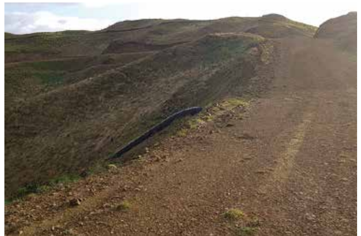
Left: The flume has good fall to reduce silting, is well pegged, and drains into slash to reduce erosion. Ribbed flumes slow water down compared with smooth bored flumes. Right: The fully flexible pipe is a good option for this exposed location
