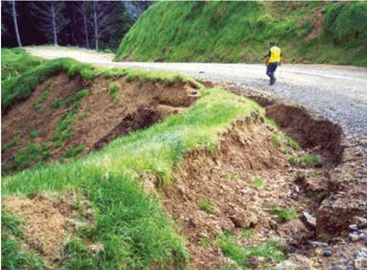
Above: An uncompacted berm vulnerable to sediment loss and failure. Right: A well-constructed berm with rock armoured ditch, hydroseeding and a slash bund at the base of the fill to contain sediment. A flumed cut out has been used to convey runoff over the fill. This berm will help protect the road and limit sedimentation
