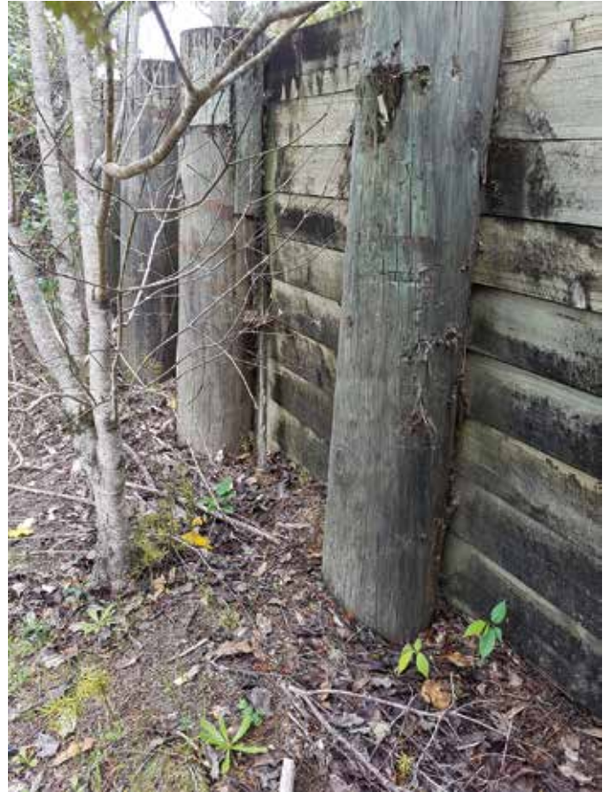
Timber cantilever retaining wall
