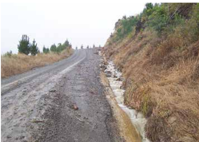
Left: A functioning ditch after heavy rain. Right: A heavily scoured ditch that has bypassed the culverts. Rock armouring and appropriate culvert spacing would have limited the impact
