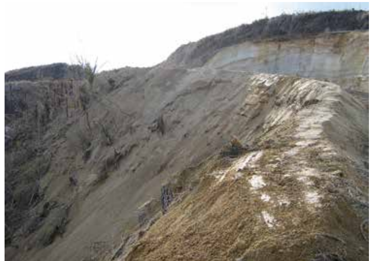
Left: Lack of a berm to control stormwater discharge over vulnerable fill has caused fill failure and sediment loss. Right: Overlarge berms create additional risk. An enlarged berm has been constructed to store excess material from cut banks. This has spilled down the fill slope to the water way in the gully. Despite compacting, the fill is now unstable and showing signs of collapse
