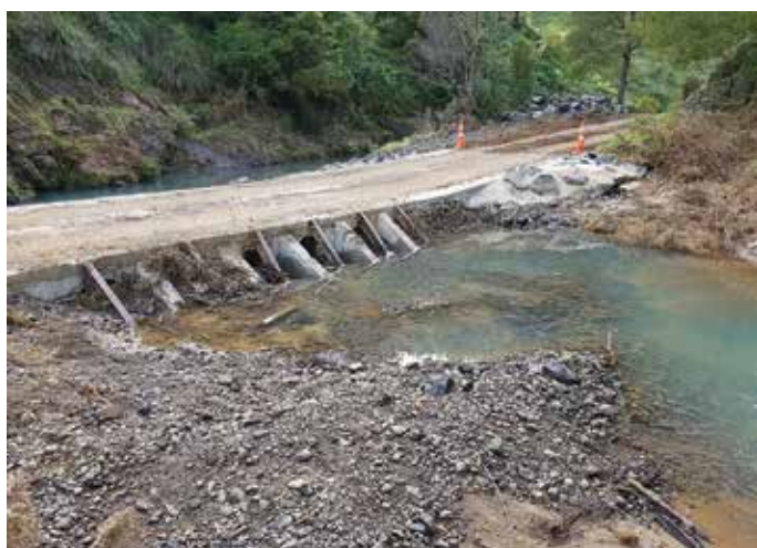
Left: The deflectors have effectively limited the amount of woody debris caught in the structure. Right: The reno mattress has protected the same crossing from being undermined, but could cause a fish passage issue if not addressed
