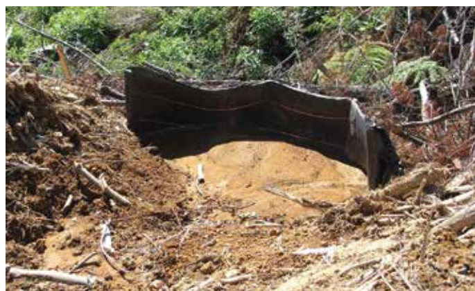
Well-functioning fences. They have captured most of the larger sediment and have not failed, despite containing a significant weight of material. Right: Maintenance is required for the shade cloth fence
