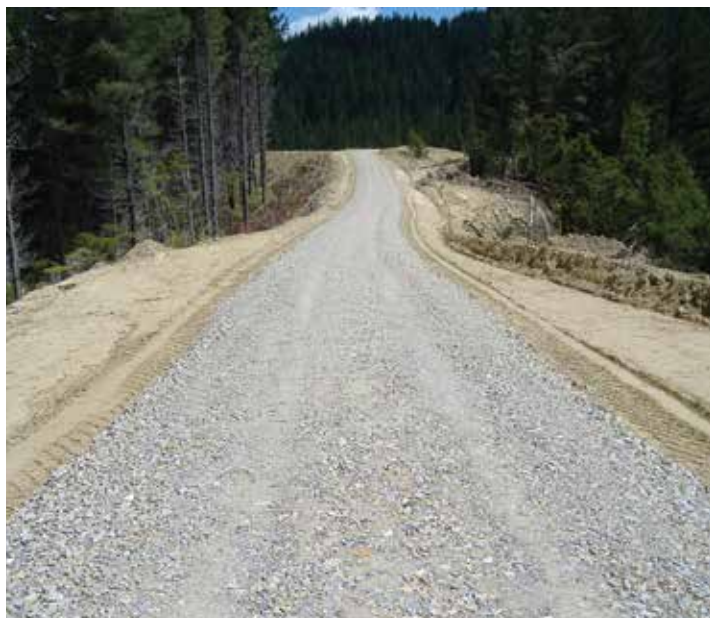
A typical one-lane secondary road. The widened shoulder on the left provides room to allow opposing traffic to pass
