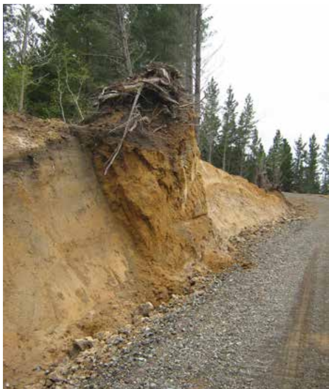
It is essential to remove all stumps prior to formation
