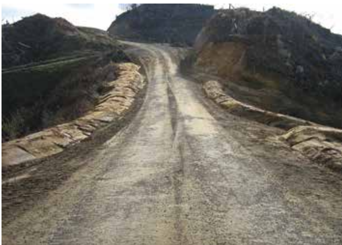
Left: Well-compacted berms were used to protect a large fill slope by directing water away from the more vulnerable earthworks. Water has been directed to cut-outs and flumes on either side of the fill. Right: This large fill is showing failure, despite having cut-outs and flumes, and will lead to environmental and access issues unless modified. The berms are too small, and the low point of the road is in the middle of a large fill slope, rather than at one end where the water can be more easily directed to original ground
