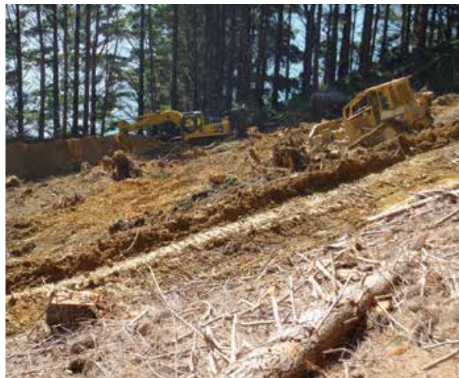
An excavator and dozer clearing and stripping
