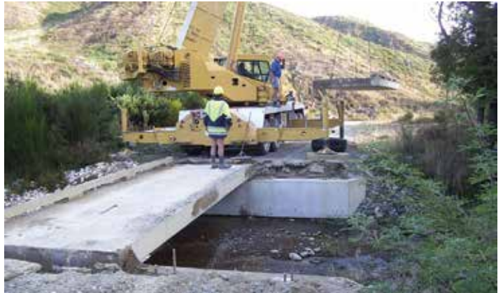
A crane will be needed to install and remove the structures
