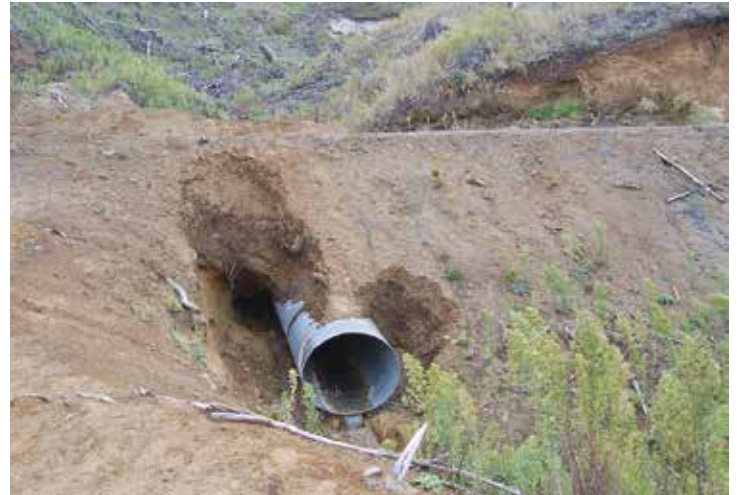
Left: Ensure provision of adequate cover of compacted fill over the pipe. Right: Poor compaction during culvert installation has led to failure as water is now bypassing the structure
