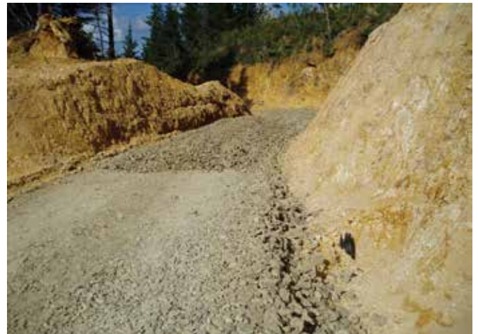
Well-graded material being placed onto the subgrade to form the improvement layer
