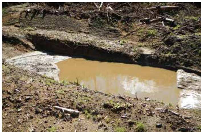
A small sediment pond. It has a low gradient cut-out to the inlet, and is constructed on the hard. It has a broad and flat, cloth-reinforced outlet to slow water
