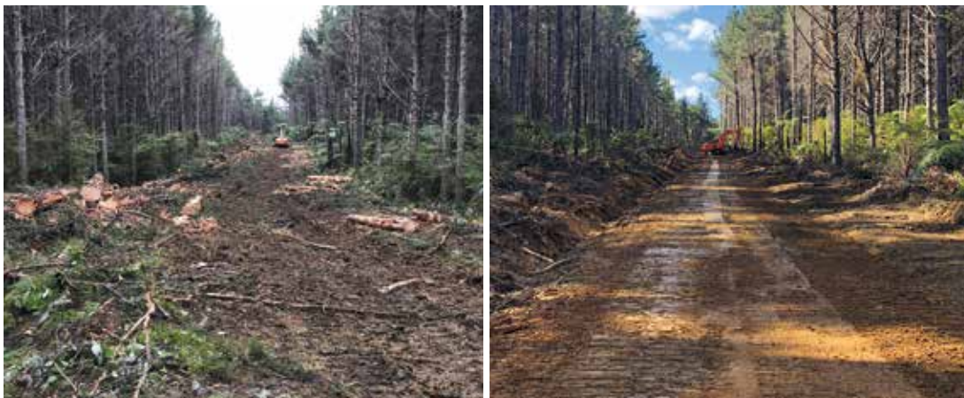
The roadline salvage width is wide enough to form the road
