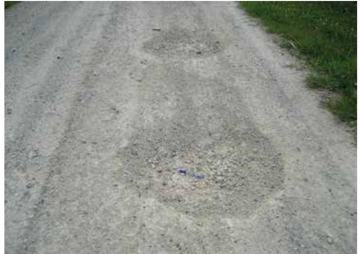
Potholes retain water that penetrates the aggregate, causing a further reduction in strength
