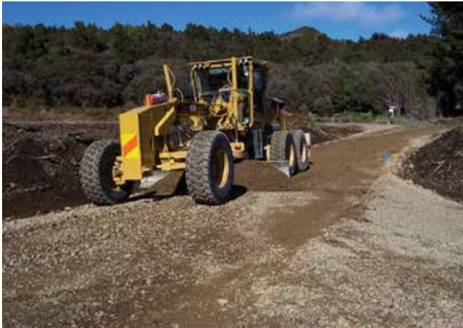
Grader reshaping road pavement
