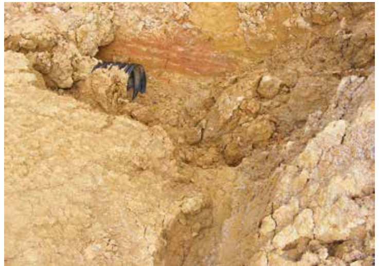
Drainage culvert mouths can easily block. Without maintenance, these culverts will likely block, and be bypassed in heavy rain. Left: Wind, not water, deposited debris has nearly blocked this culvert. Right: Bank collapse and sediment infill is a common issue
