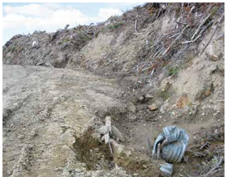
Check for crushed drainage culverts after logging. Drainage culverts are easily damaged if the maintenance operator is inattentive
