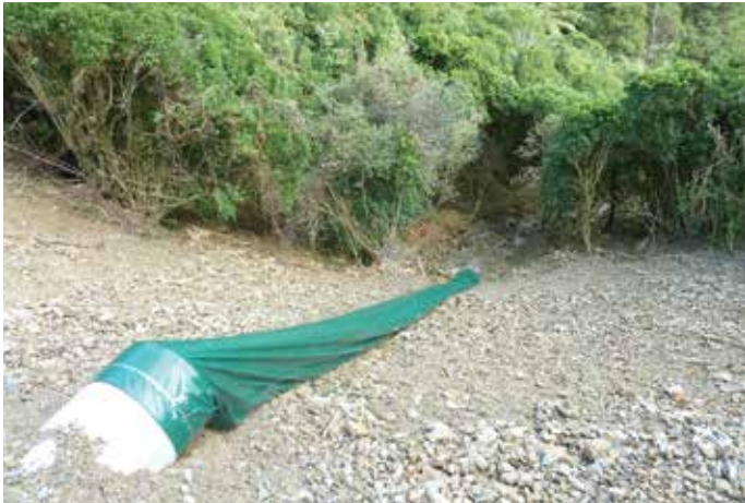
Left: Culvert sock securely attached to culvert and anchored. Right: A poorly designed and secured sock; the inlet has been bypassed and the wind has twisted it
