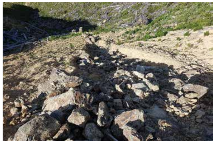
Left: Galvanised iron or tin flumes are not good practice. They increase water speed, and cannot easily follow the terrain. The sheets do not lock together, and can fall apart. Right: Rock armouring cut-outs and culvert exits are an effective way to reduce water speed and scouring
