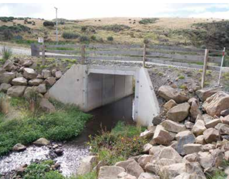
Example of a large concrete box culvert
