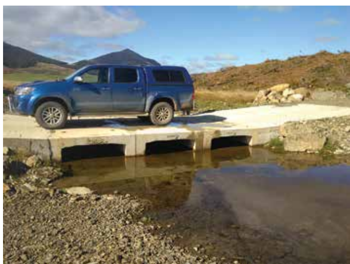
Left: A well-constructed drift deck. Right: A drift deck crossing, with a secondary crossing for tracked logging machines that would damage the concrete pad
