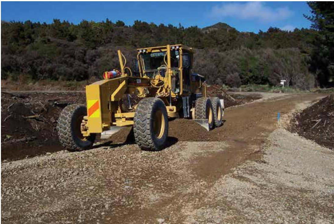
A grader is used to spread the pavement layer over the newly formed road. This layer, when compacted correctly, will provide a good, strong running surface and prevent moisture from infiltrating through to the base course or subgrade layers
