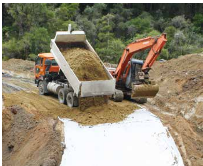
Geosynthetic cloth being used as a separation layer
