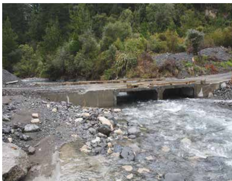
Left: Drift deck outflanked by the river. (Credit: D. Nielson). Right: Drift deck components ready for installation
