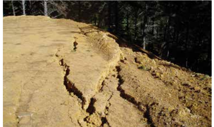
Left: While side casting is often the easiest way to build a road, the material pushed over the edge onto the slope is very susceptible to erosion and failure. Right: Tension cracks have developed on the landing. Over time it will allow water to infiltrate and cause the fill slope to slump. It is very important to correctly bench and compact fill material
