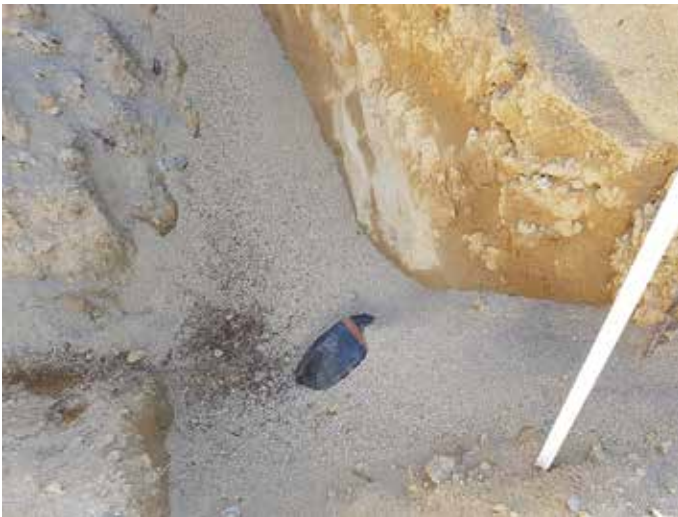
Drainage culvert mouths can easily block. Without maintenance, these culverts will likely block, and be bypassed in heavy rain. Left: Wind, not water, deposited debris has nearly blocked this culvert. Right: Bank collapse and sediment infill is a common issue
