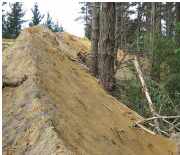
Left: Well-marked road clearing limits. Right: The clearing limits were not marked wide enough
