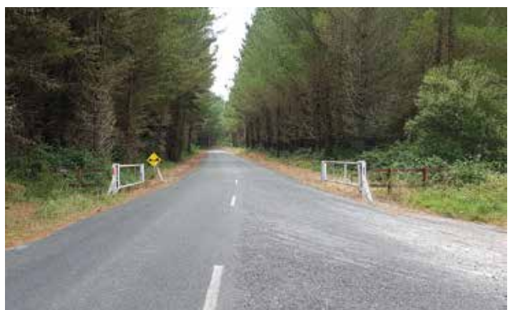
A sealed forest arterial road
