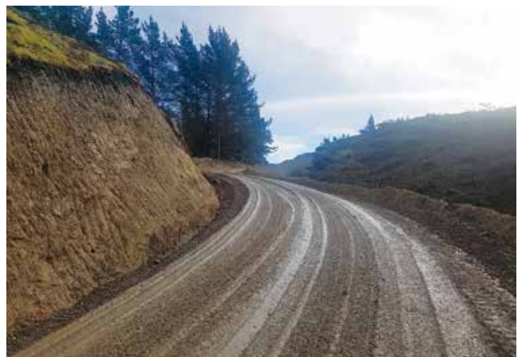
Left: Scouring can rapidly occur during heavy rain. Right: Good crossfall helps reduce scouring
