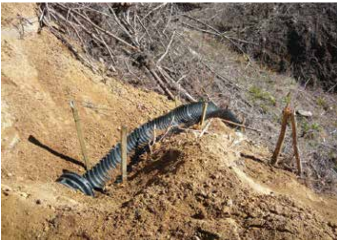
Left: The flume has good fall to reduce silting, is well pegged, and drains into slash to reduce erosion. Ribbed flumes slow water down compared with smooth bored flumes. Right: The fully flexible pipe is a good option for this exposed location
