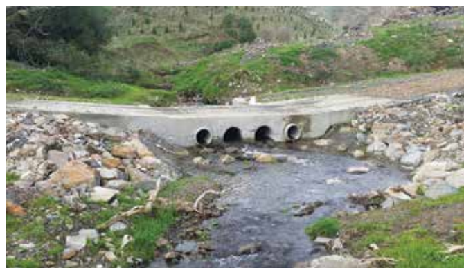
Battery culverts must provide for the river's base flow, and upstream and downstream passage of fish; one pipe must be buried 100 mm into the river bed
