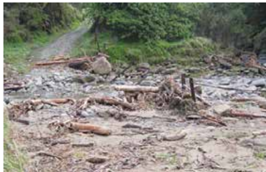
Left: Radiata stumps are not preferred anchors, as many will have lose their tensile strength within the design life of the structure. Right: There was too much energy in the river and the structure failed. The storm flow moved large boulders, as can be seen of the far river bank. Consider putting traps in side creeks or where the river's energy lowers
