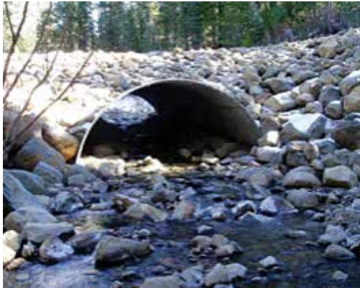
An arch culvert that maintains the natural channel substrate
