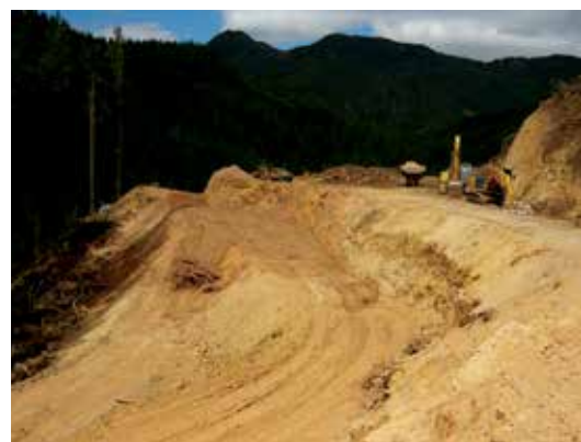
Above: Balancing cuts and fills help minimise the overall earthworks required to construct a forest road Below: Landings can generate large volumes of earthworks. Benching is essential in anything other than the easiest country to help stabilise the fill
