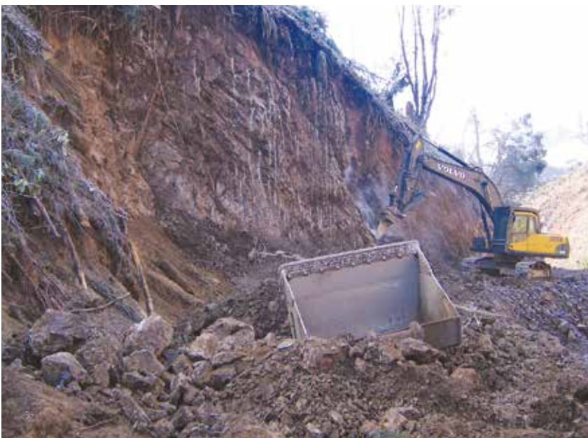
Severe low production digging with a single ripper tine smoking away
