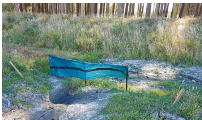
Left: Sediment fences are not designed for watercourses. They fill rapidly, divert flow, or fail. Right: This fence is inadequate. The lower edge has not been buried properly, so has blown out. The fence is not wide enough, and there are no wings so stormwater flow would have bypassed it. Also, it is too close to the waterway immediately behind it
