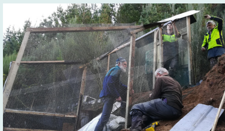
Installation of the predator fence
